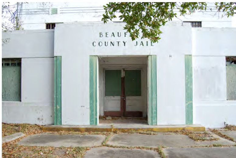
▲ EXISTING JAIL BUILDING
