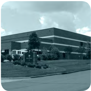
Industrial, warehouse, or distribution-type building
